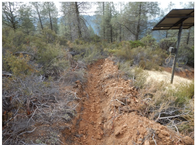
Photo 4 (Magnuson) - Drainage around OC1 (Facing South)
