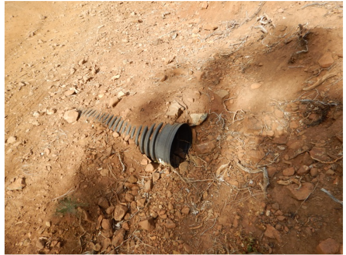
Photo 14 (White) – Crossing C3
