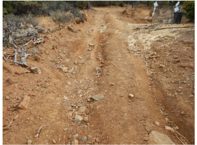
Photo 8 -Downslope of OC3(Facing Northeast)
