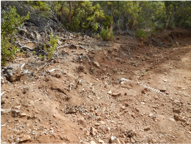
Photo 13 (Magnuson) – Crossing C3 (Facing East)
